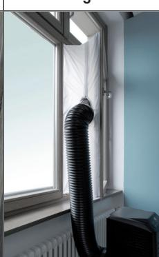
A wider photograph showing the window fully open. A black flexible exhaust duct is connected to the window frame, passing through a circular hole. The duct is connected to a white rectangular device, likely a fan or air outlet, which is resting on a radiator below the window. |
