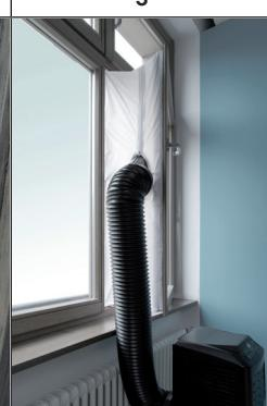
A wider photograph showing the window fully open. A black flexible extraction duct is connected to the bottom of the window frame. The velcro strip from the previous steps is visible at the top of the frame, sealing the gap between the window frame and the duct. |
