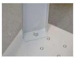
Bolt the lower ends of the collector support to the base plate using M8 x 16mm hex head bolts and M8 washers.
