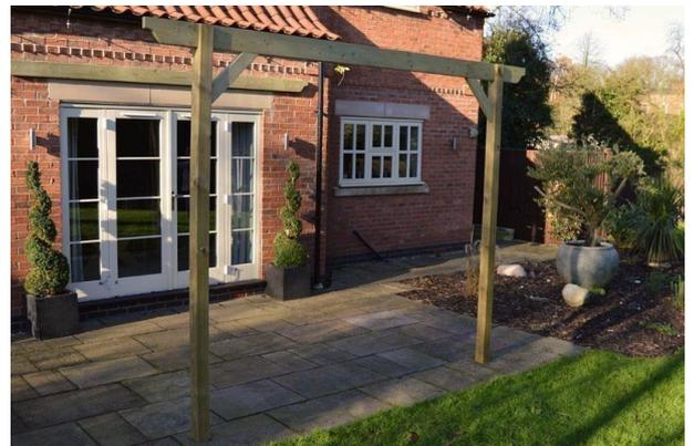
Now stand the end frame up vertically as shown using 2 assistants and manoeuvre it into place so that it is wood approximately in place, parallel to and about the length of a rafter away from the wall plate.
