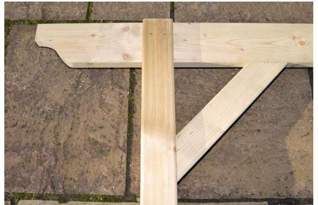
Place one of the diagonal braces (500mm) in place, adjusting the post angle if necessary, so that it butts snugly up to the inner edge of the runner and post. This ensures that it is set at 90°.
