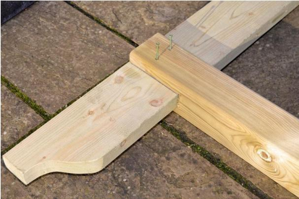
Now slot the remaining runner into the top of the post as shown using the pencil mark to align the runner with the outer edge of the post. **Please note both sides of the runner must have the overhang of 40.5 cm.**
