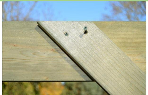
Now, add the longer braces (800mm) to the frame. Align top with the top edge of the rafter. Make sure that, bottom face of the brace is flush to the post. Secure with provide shorter wood screws. Repeat this step for both sides.
