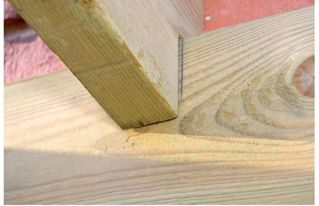
Make sure that the other end is aligned between the pencil marks on the wall plate. If necessary, adjust the position of the end frame to get everything square and properly positioned.
