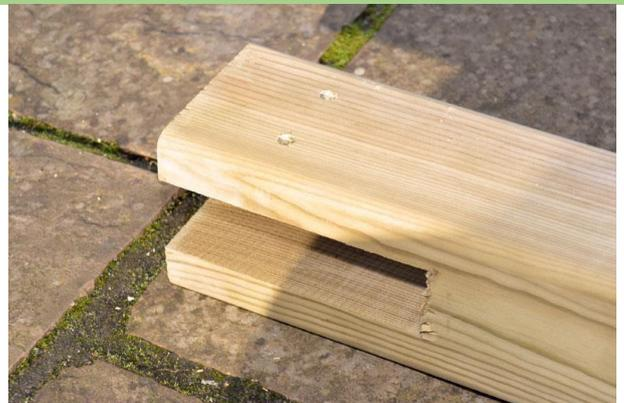
Lay down one of the posts with the slot parallel to the ground as shown.
